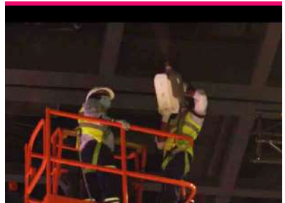
Air change rate in the halls is 8 times per hour. Air extraction in the halls is pre-scheduled and all hall shutter doors will be kept open both before and after the event to assist with air circulation
